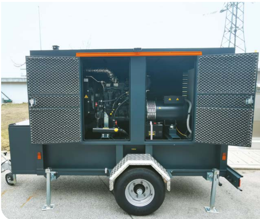
60 kVA mobile power generator
