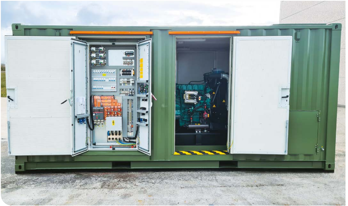
"OHMEGA" 250 kVA emergency power supply
